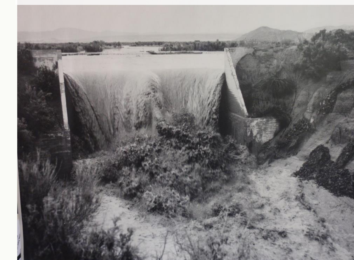
1940 – working hard to trap sediment and hold the Panaca Meadows in place
