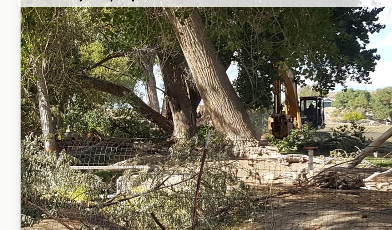
Heavy equipment used to clean the Drain
